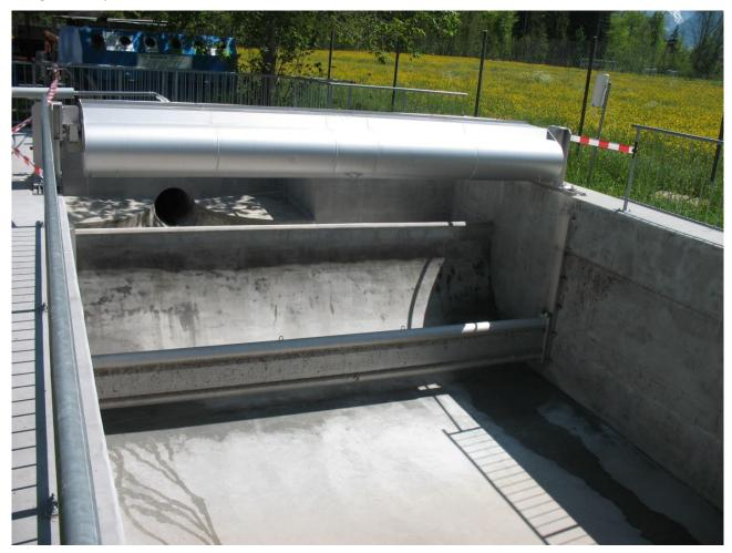
Figure 2: Flushing dump in the open basin
