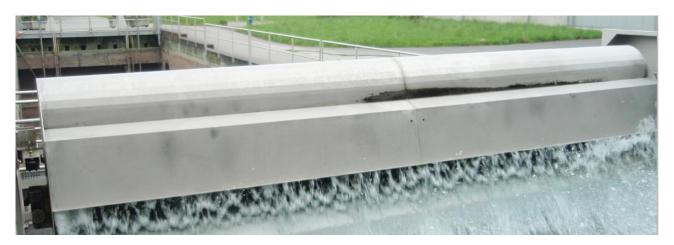
Figure 1: Flushing dump
