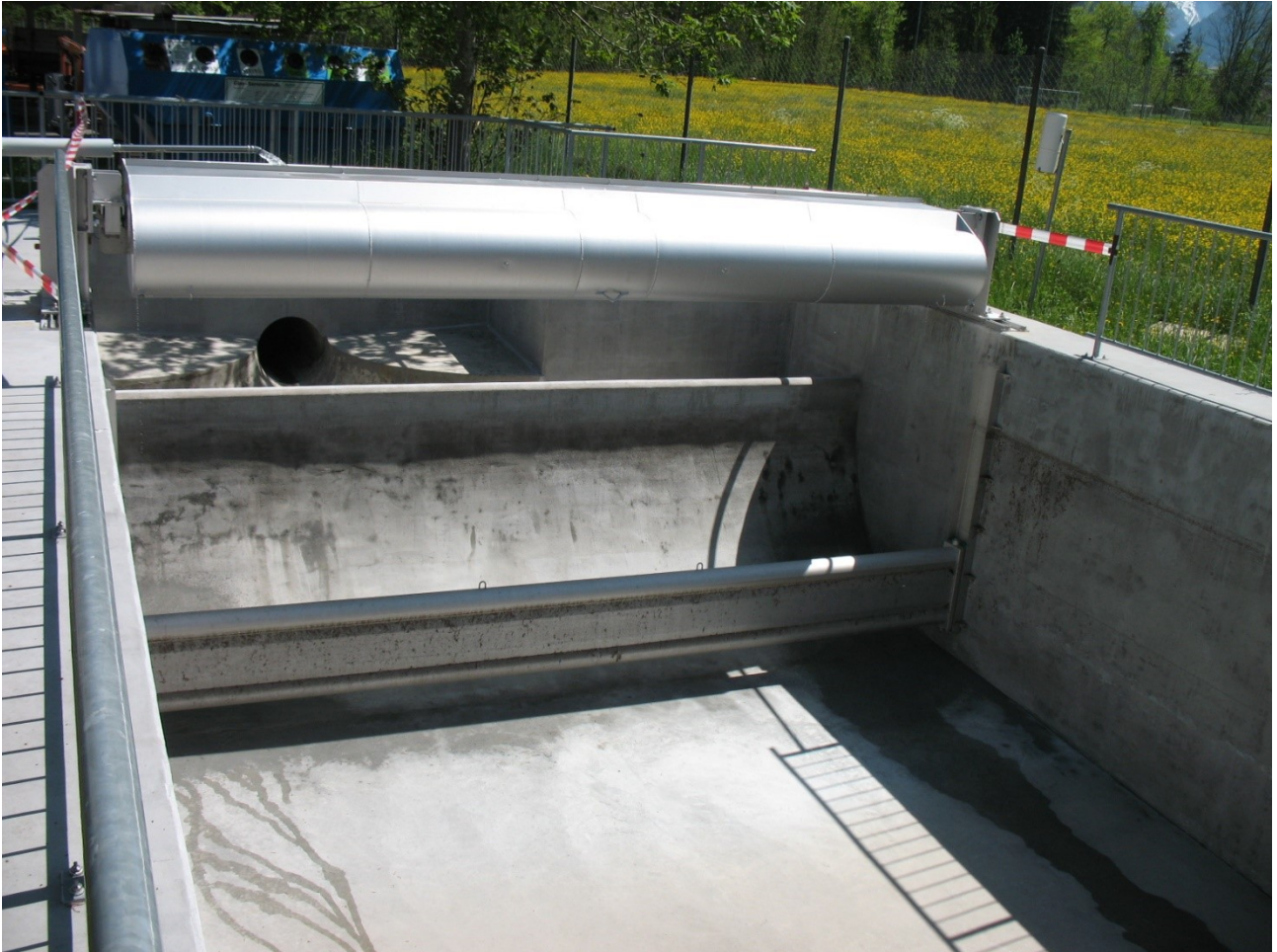
Figure 2: Baffle in the open basin
