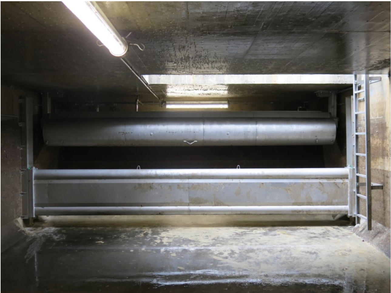
Figure 1: Vertical floating scum baffle
