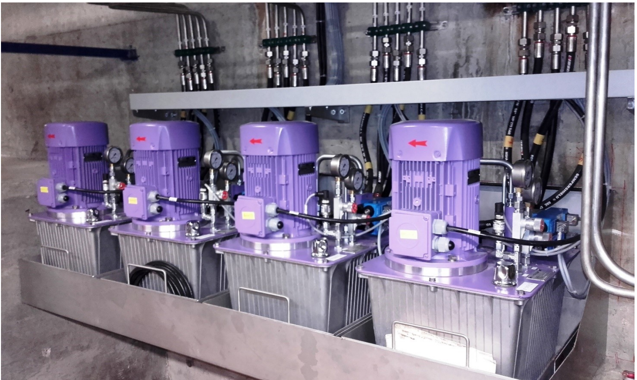
Figure 7: Hydraulic system for multiple screens
