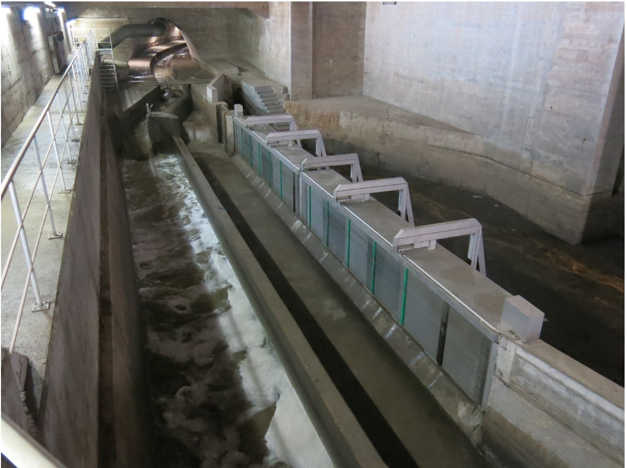
Figure 5: Vertical screen with special arrangement in Lausanne, Capelard.
