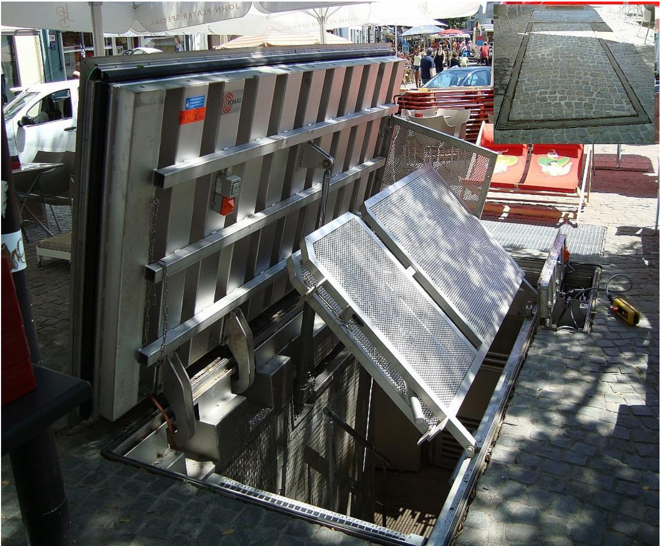
Figure 2: View construction / installation
