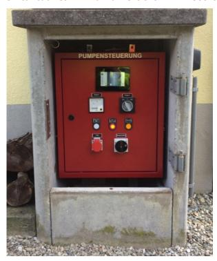
Figure 6: ALLinONE for 1 wastewater pump using the example pumping station in Meiringen BE/CH; Cabinet WxHxD 500x600x250mm retrofitted in an existing concrete cabin.
