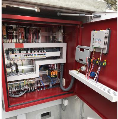
Figure 8: ALLinONE interior using the example of the Dättnau stormwater tank of the city of Winterthur; cabinet WxHxD 1000x800x300mm incl. space reserves.
