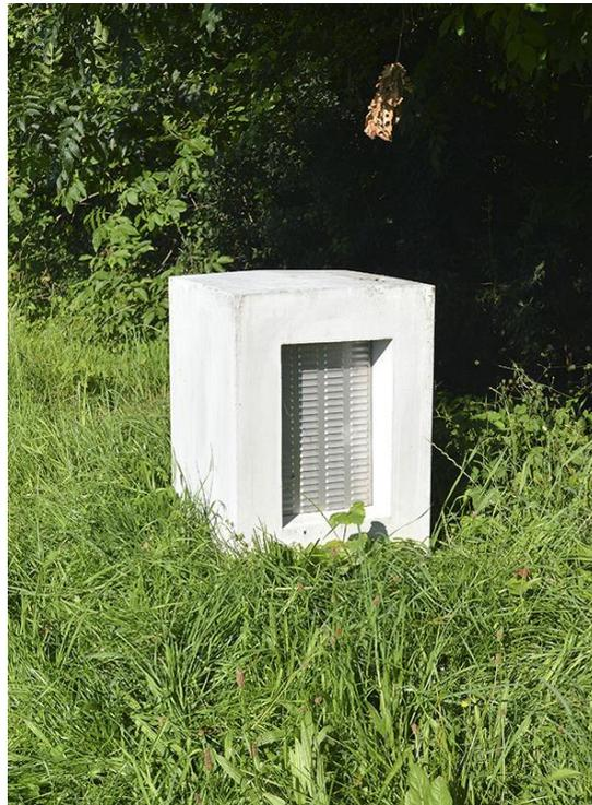
The massive exhaust boxes of concrete provide efficient protection from vandalism.
