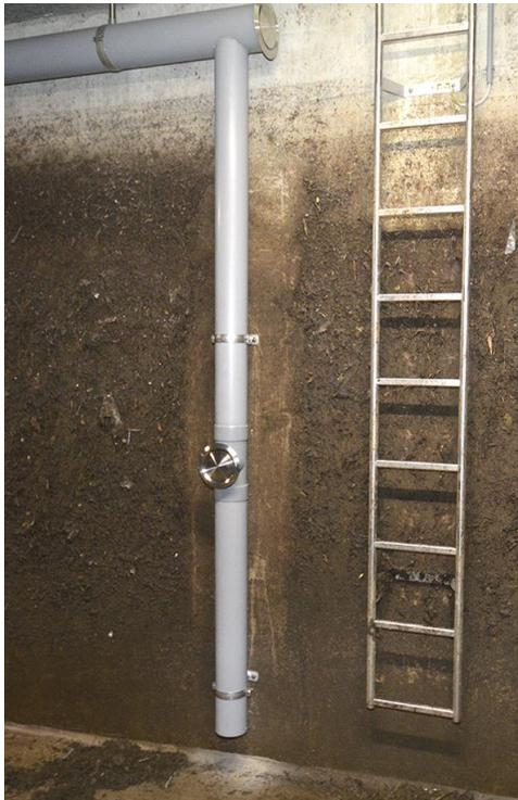
Depending on the water level, the air is exhausted at different heights: right at the bottom, on the level of the metal cap or up under the ceiling.
