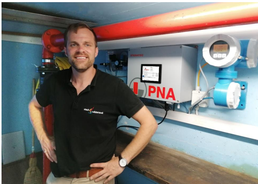
Figure 2; Fritz Seewer, Project Manager Civil Engineering Office of the City of Wädenswil in front of the latest control of one of his MID-controlled PNA flow controllers.
