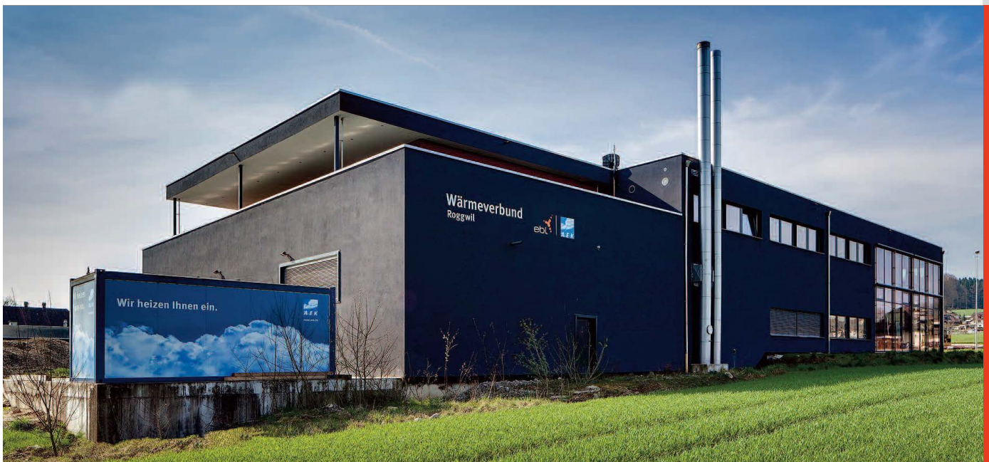
The district heating center in Roggwil, one of the plants managed by the AEK Energie AG, which is integrated in the STEBalarm alarm system.
