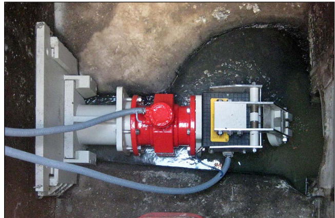
afterwards Size NW 200 pneumatic outflow control with two-part installation adaption
