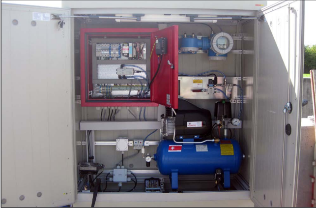
Compact free-field control cabinet with ventilation, heating, air compressor, control unit with touch control and emergency throttle
