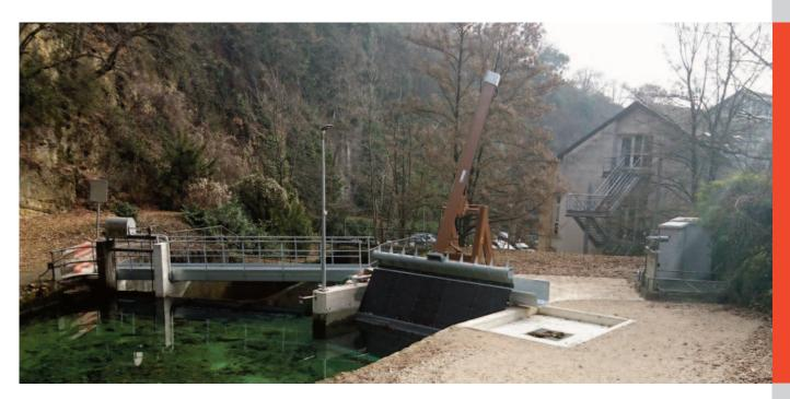
The new plant at a glance (starting from left): Overflow gate, lighting, screen cleaning machine with screen array, flushing conduit and concrete tub, main gate and concrete booths for hydraulic unit and control cabinet.
