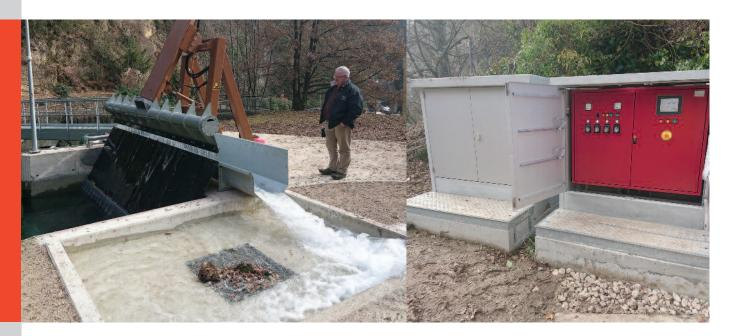
The floating trash, which the cleaning machine lifts into the flushing conduit, is flushed into the concrete basin with bottom screen.
