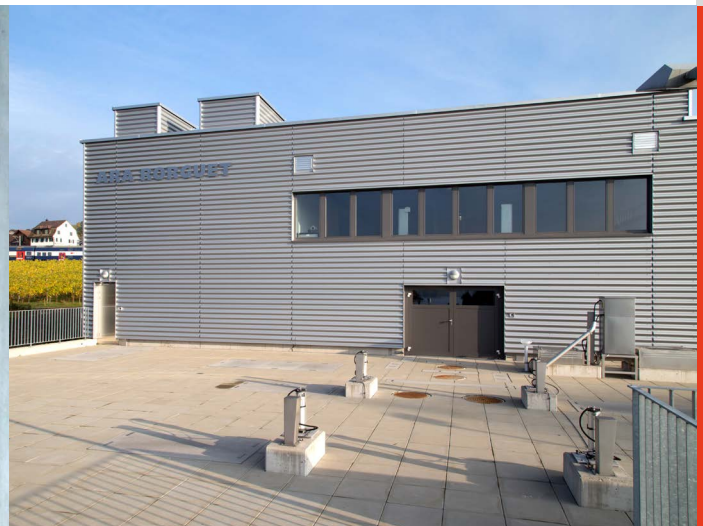
The Rorguet waste water treatment plant treats the waste water of the three municipalities Meilen, Herrliberg and Uetikon am See.
