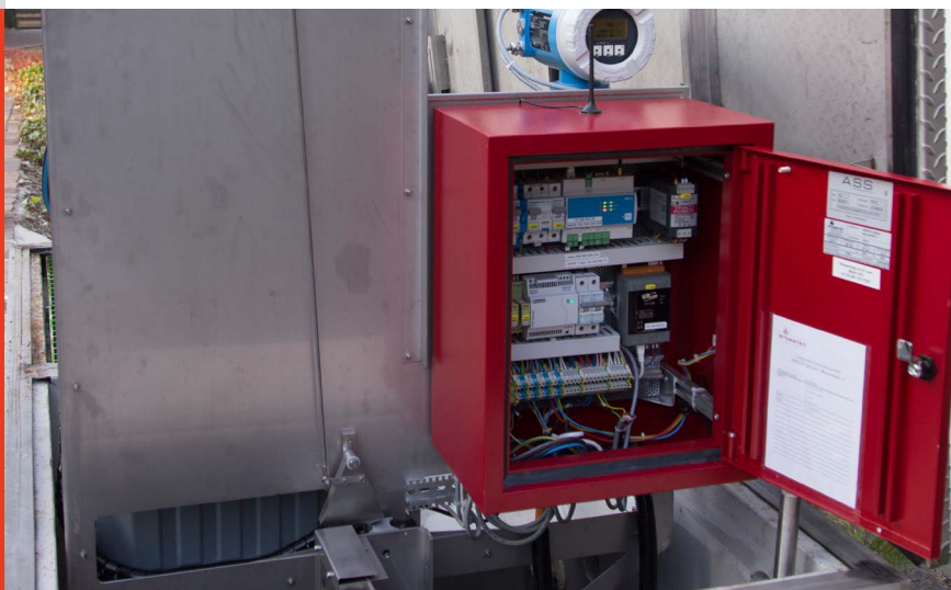
Access to the control cabinet is unobstructed.
