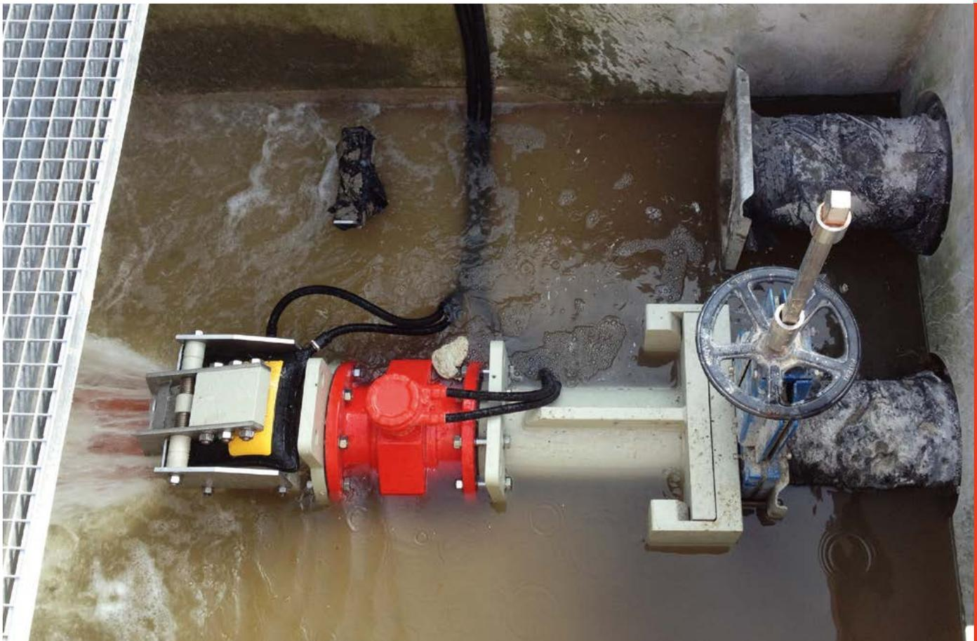
The Oberregenbach sewage treatment plant of the town of Langenburg (D) is located between Stuttgart and Nürnberg and treats the waste water of about 1,800 inhabitants. Located on the foot of a slope, the water from the storm-water basin runs down a steep canal. Before the STEBATEC drain controller was installed, the waste water was slowed down by a mechanical scale throttle before it entered the sewage treatment plant.
