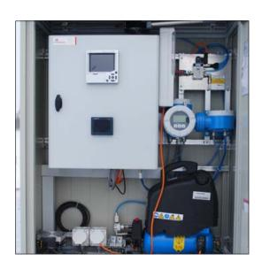
Free-field aluminum cabinet for pneumatic outflow control.
