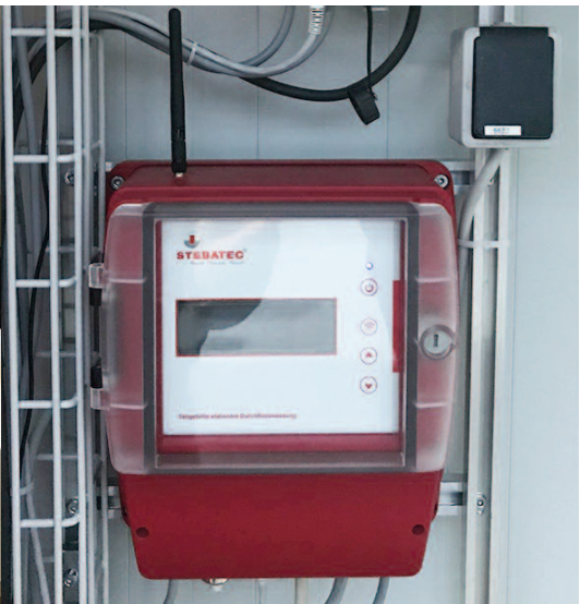
The measuring transducer from Stebatec transmits flow data to the SCADA system or optionally to other users via GPRS.
