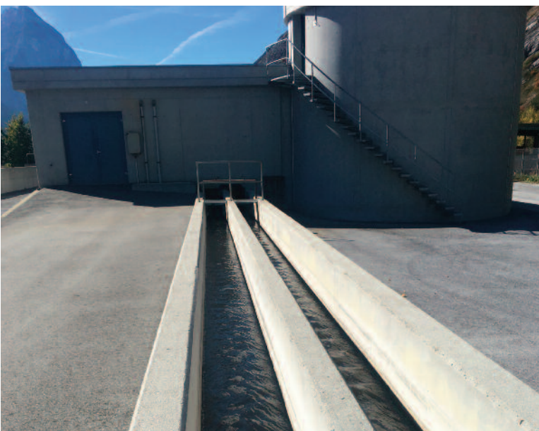
With the overflow measurement, the Radet waste water treatment plant can now reliably determine the inflow during rainy period.
