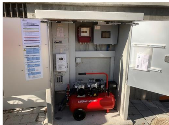
Figure 5: The system was purchased from STEBATEC including cabin, compressed air treatment and data transmission to the sewage treatment plant.
