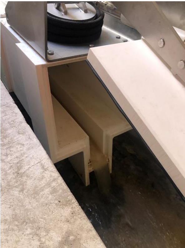
Figure 2: Outlet area of the TF-PNA. During dry weather the throttle valve remains open while the small discharge quantities in the dry weather gutter are precisely measured.
