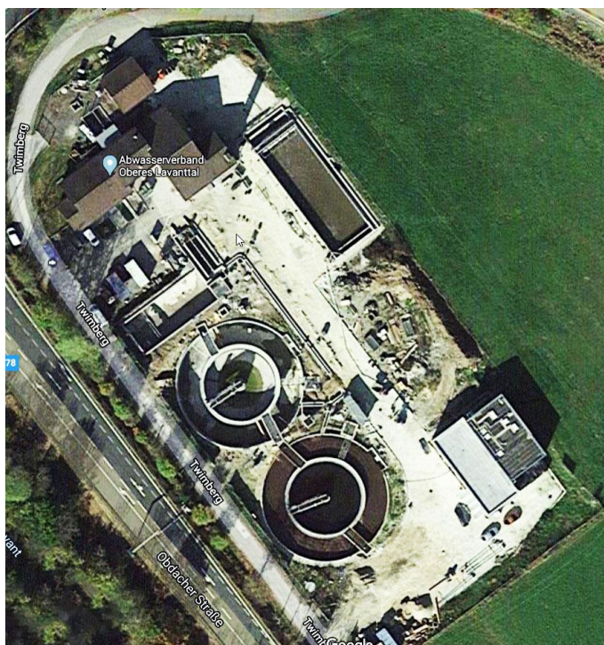
Figure 2: Overview Twimberg wastewater treatment plant
