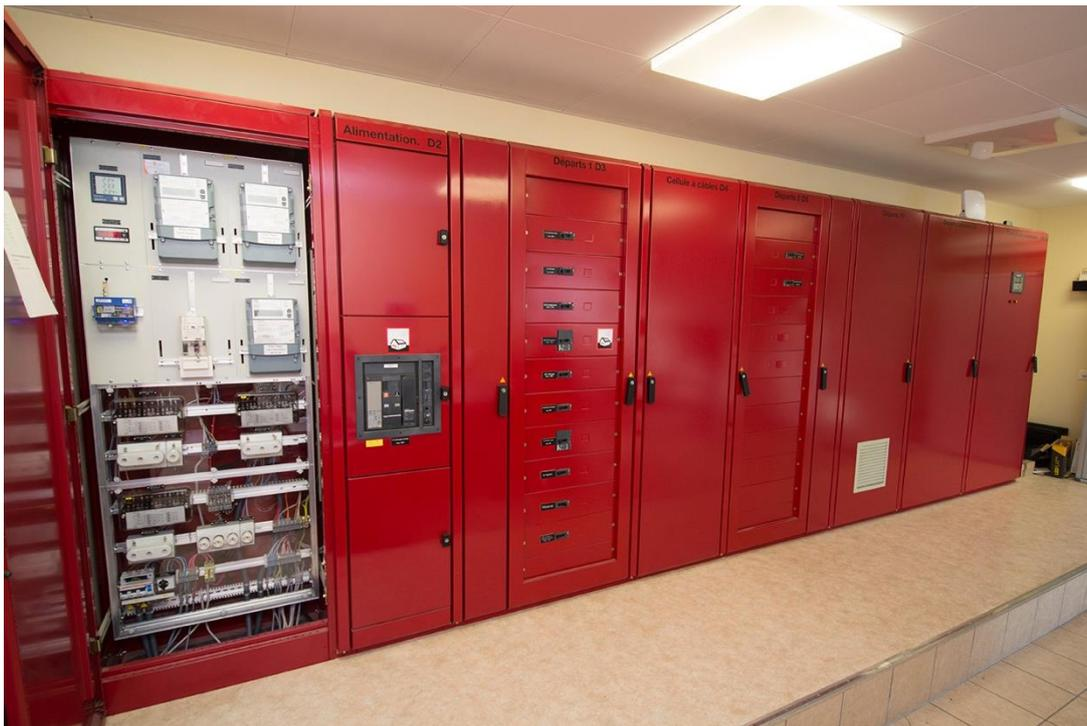
The electrical circuits were partly renewed and supplemented by emergency operation decoupled from the public grid.
