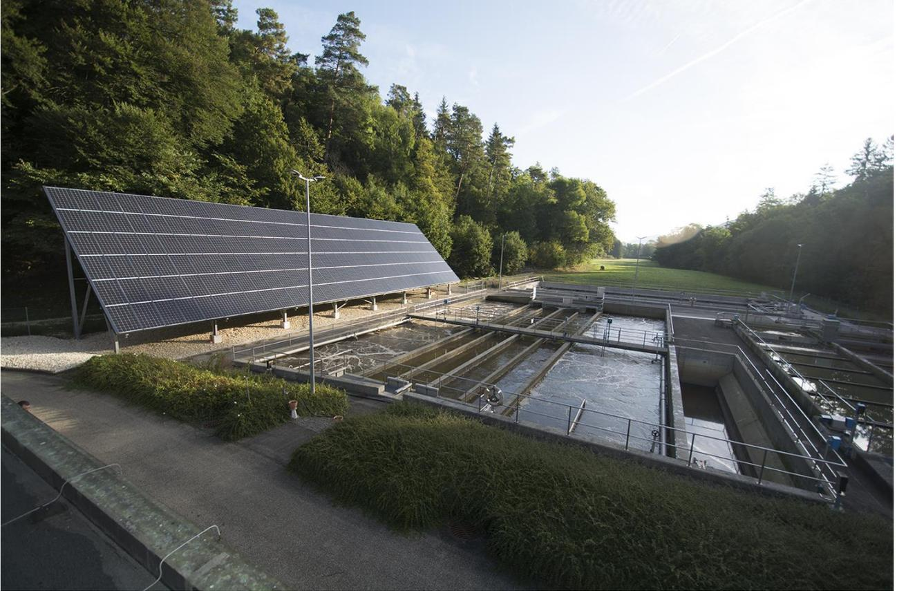
The new photovoltaic system is designed to cover at least 10 percent of the electricity consumption of the WWTP even in bad weather.
