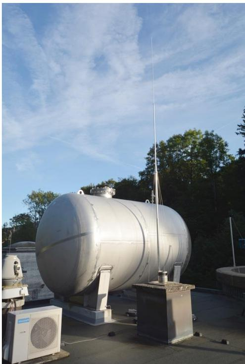
The additional gas tank triples the storage volume and thus creates greater flexibility. The antenna is used for lightning protection.
