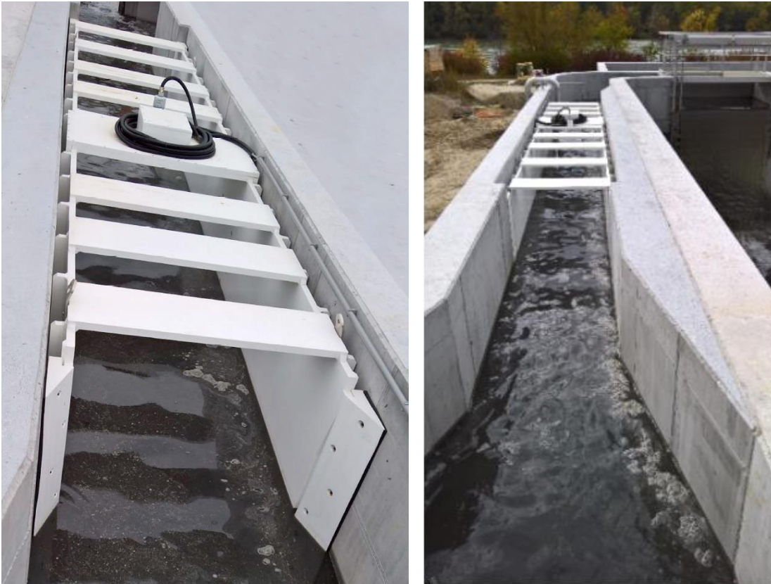
Figure 1: View after conversion
